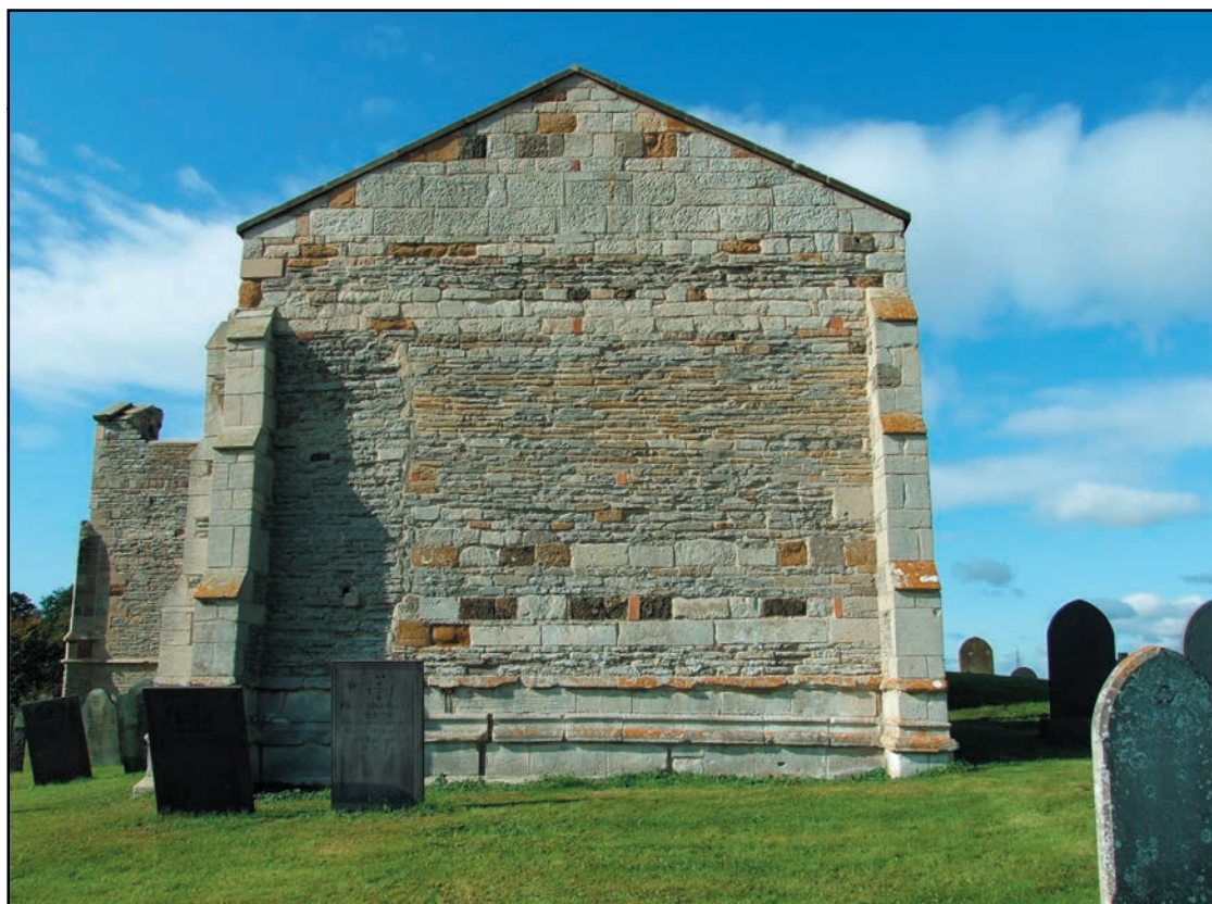
Figure 17. The east wall, rebuilt without a window.
