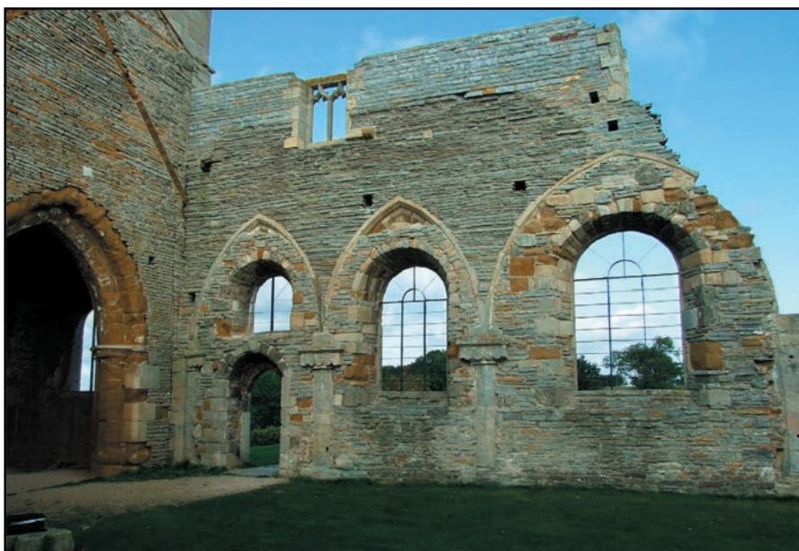
Figure 7. North Arcade Nave Wall. The two and a half rounded columns with scalloped capitals, all Lincolnshire Limestone, are typically Norman. Subsequently the North Isle was raised with the insertion of ribbed pointed arches mostly oolite with some sandstone. The first two are set below the ironstone roof rib of the tower, but the third is taller and wider. Georgian style windows were inserted when the arcade became the Nave Wall.
