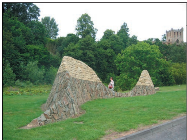
Figure 6. James Hutton's memorial wall at Jedburgh, with sandstone above and greywacke below.
