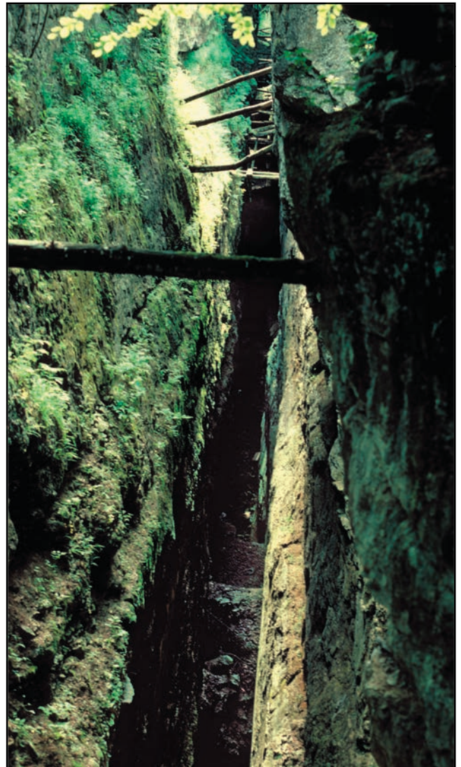
A sight now lost - the view west along the open stope on Long Rake as it was in the late 1970s. The opening was about 5 m wide, and here about 30 m deep, though the visible floor was formed by piles of waste "deads" stacked on timber platforms above open stopes that descended another 60 m or so.
