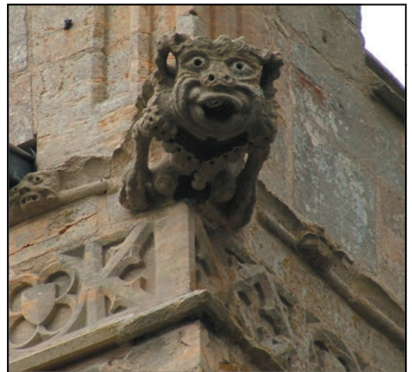
Figure 13. Gargoyle at SW corner of Tower, set above a carved frieze, both in Lincolnshire Limestone.
