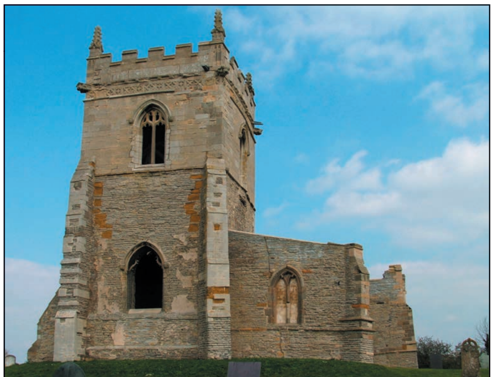
Figure 1. The surviving remnants of the walls and stonework at St Mary's Church, seen from the west, on its low hill northwest of the village of Colston Bassett.
