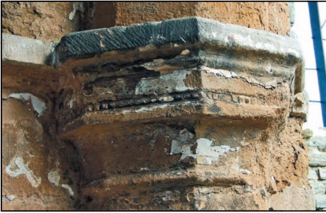
Figure 10. Nailhead decoration on the capitals of a column supporting the Tower's arches, with traces of old whitewash.
